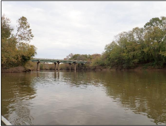
Image 4. The bridge over the Staunton River for Route 360 (James D. Hagood Highway/Kings Highway).
